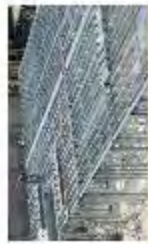
Framing 2"x6"16ga Cold Formed Framing
